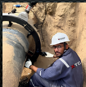
Pipe Cold Cutting
